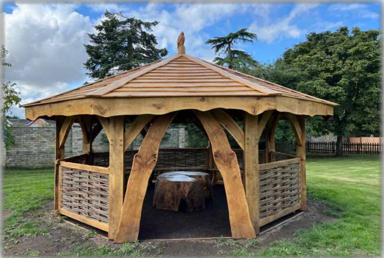
The Octagon at Kings School Ely. Built around the stump of a much loved 250 year old oak tree, with much of its timber milled from the trunk.
