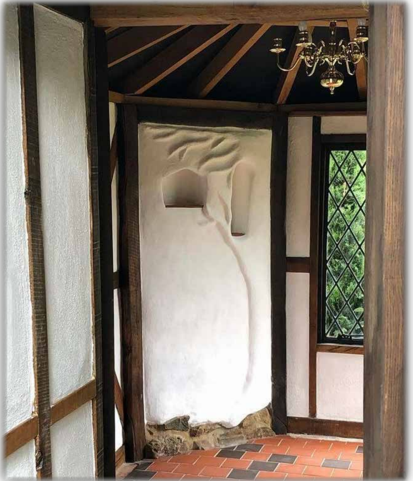
An example of how cob can be used to create stunning feature walls. We finished this piece with clay render and lime paint.
