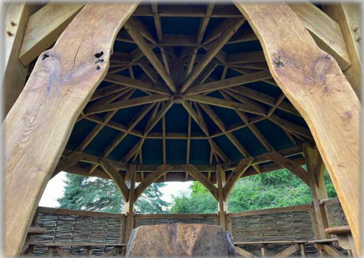
The Octagon at Kings School Ely. Built around the stump of a much loved 250 year old oak tree, with much of its timber milled from the trunk.
